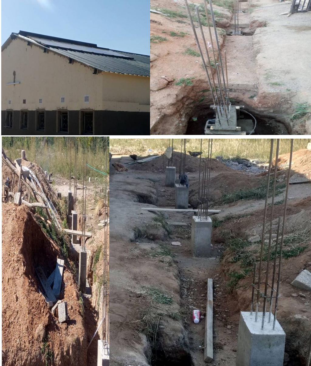
Casting of the ambulance bay reinforced concrete columns.
